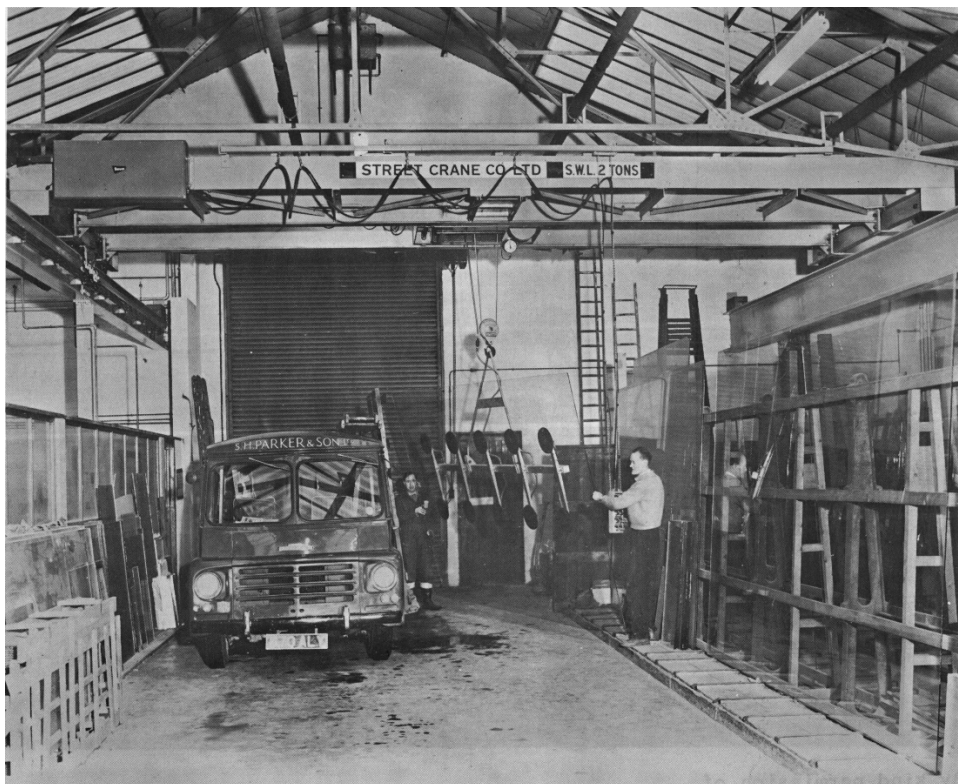
Glass handling crane with vacuum lifting frame circa 1962
